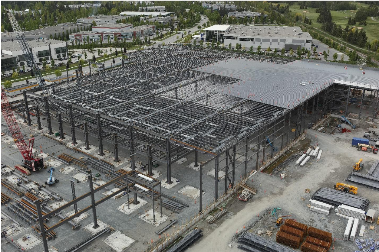
Figure 1: Aerial view of steel-frame warehouse where incident occurred.
