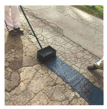
Spalding County also uses a Crafco Patcher II melter, a double-boiler unit that's specifically designed for mastics. The unit's digital controls maintain proper material application temperature and mixture to make it easy for the crew and ensure a successful repair.
