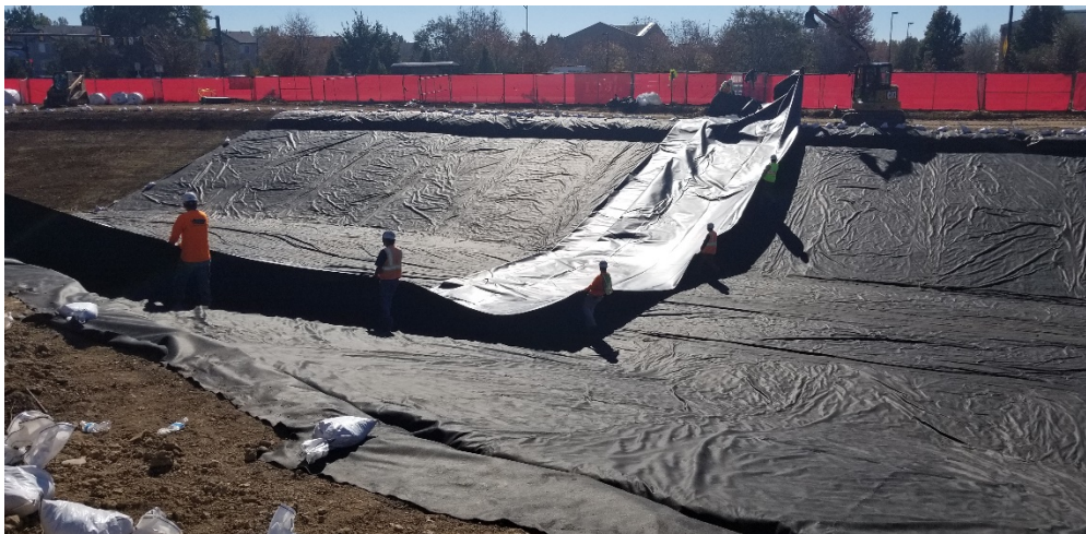
Installation of the new pond liner
