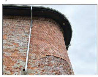
It's clear to see where the new brick has been used, and the new roof designed to help water run off and away from the fort.
