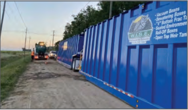
Ten frac tanks held the contents pumped from the Cole Drain until it could be pumped away. (Screenshot)
