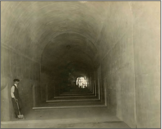
The scale and engineering of the Welland Ship Canal is displayed in this photo of a canal construction worker standing in the large sluice tunnels on the inside of the lock walls.
