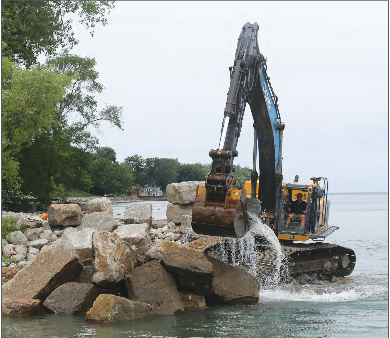
In March, a storm washed away some of the bottom below the large anchor stones, and one was completely washed away. In February, 2020, Dock Area resident Ron Simkus had warned of just such an incident. The town had repairs done in June to make the groyne safe, and will take the next month to decide what to do next. (Photo supplied)
