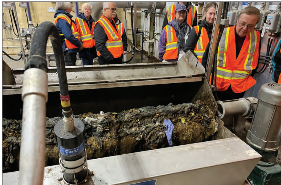
Tour participants take a look at the mechanical bar screen that picks out large solid items from the wastewater early in the process after it arrives at the Port Weller Wastewater Treatment Plant.
