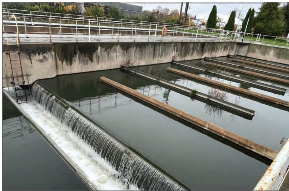
The final step in the clarification process as gravity feeds the clean water into Lake Ontario.
