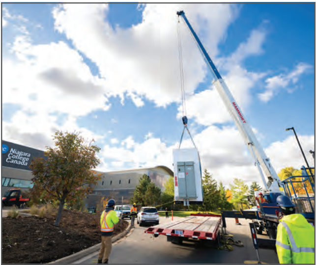
A crane from NOTL Hydro lifts an industrial battery for energy storage on to the NOTL campus of Niagara College. (Supplied)
