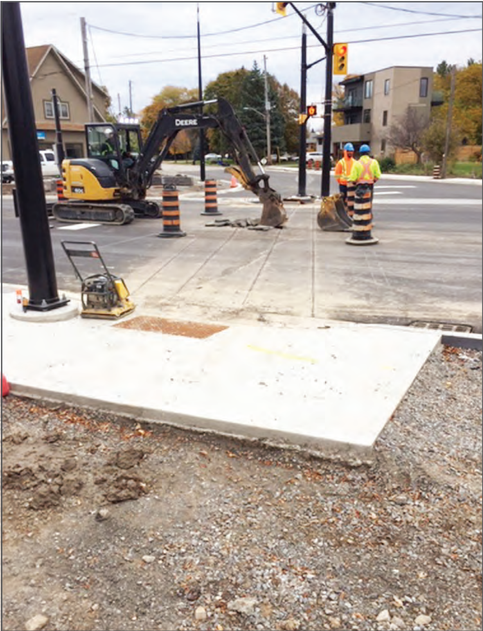
This photo shows pavement completed and torn up — for a good reason. It allowed for decorative pedestrian crosswalks to be installed at Field Road and at Line 1. (Supplied)
