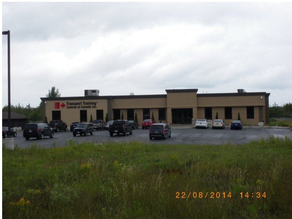
PHOTO 3 2565 KINGSWAY, SOUTH OF THE SUBJECT LANDS VIEWED LOOKING SOUTH FROM THE KINGSWAY
