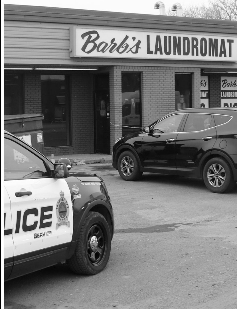
LOOKING INTO IT: Police were called to a fire early Sunday morning at Barb's Laundromat on Cumberland Street. No one was injured in the fire, but the business suffered heavy damage.
