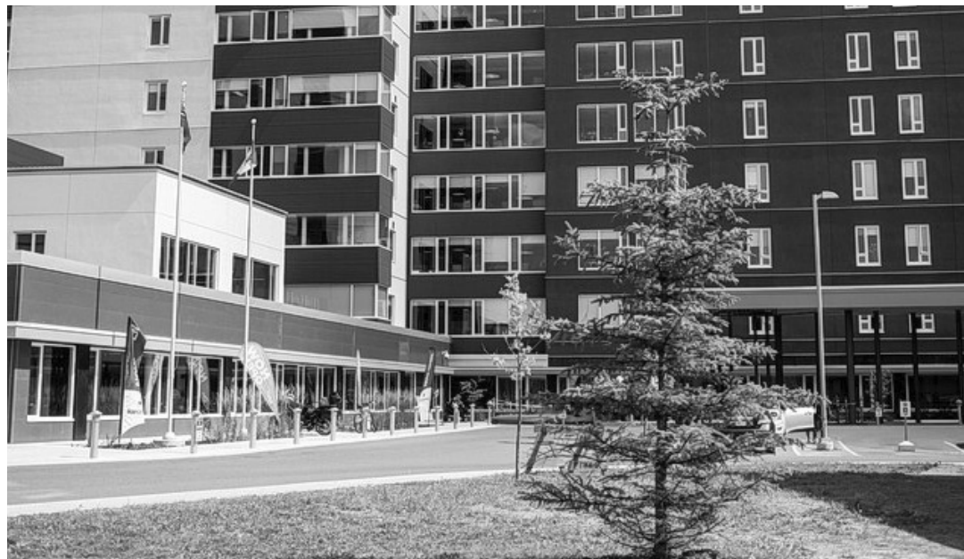
STAYING SAFE: Precautions have been put in place at Hogarth Riverview Manor after a positive COVID-19 test.
