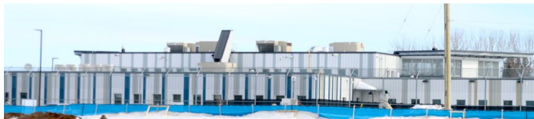
CORRECTIONAL EXPANSION: The 50-bed expansion to the Thunder Bay Correctional Centre is now housing inmates.
