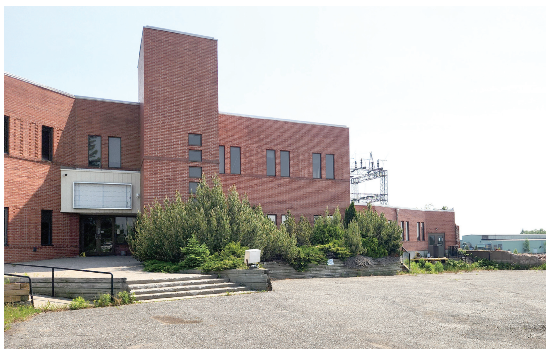
A proposed lithium-hydroxide processing plant could be built on the site of the former Abitibi pulp and paper site. (Gary Rinne)
