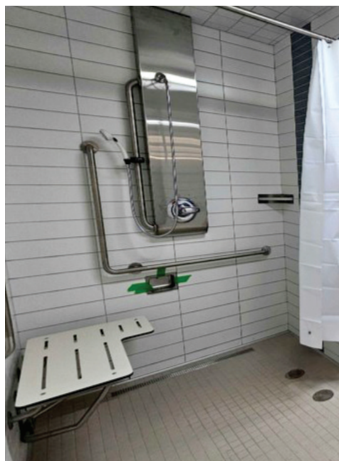
An accessible shower in the men's changing room.
