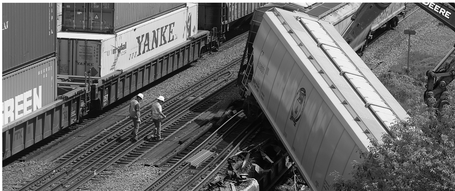
OFF THE TRACKS: A Canadian Pacific Railway train partially derailed on Tuesday, one car jumping the tracks at the bridge over McVicar Creek.
