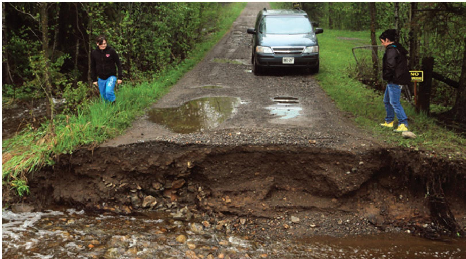
UNDER WATER: Road washouts were a common sight in May 2012 when a torrent of rain led to flooding throughout the Thunder Bay area, including a water treatment plant failure.
