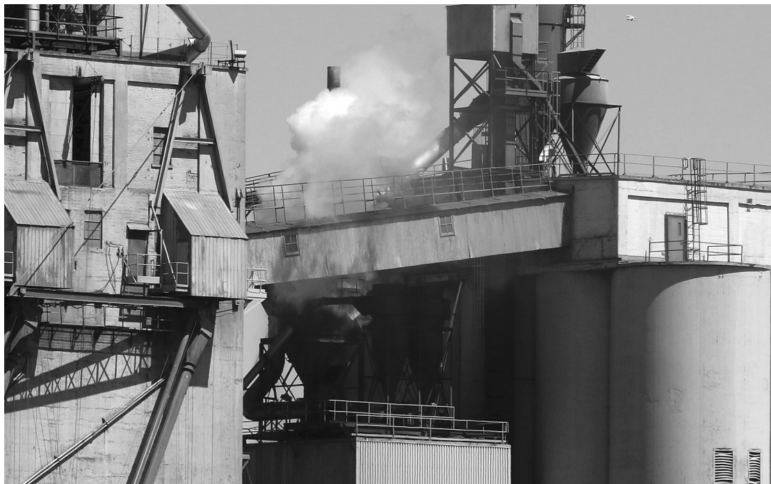
UNDER CONTROL: Thunder Bay Fire Rescue say no one was hurt in a Sunday afternoon fire at a pellet plant at Richardson Terminals.
